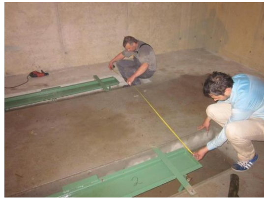
Image 3.4: Installation de la structure
